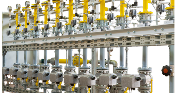
Mixing system in the glass industry
